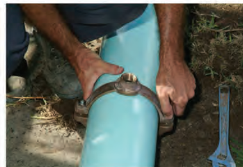
Figure 7.12: Most tapping bands providing full circle support to the pipe are suitable for ApolloBLUE™. A Milnes gunmetal band is shown here.
