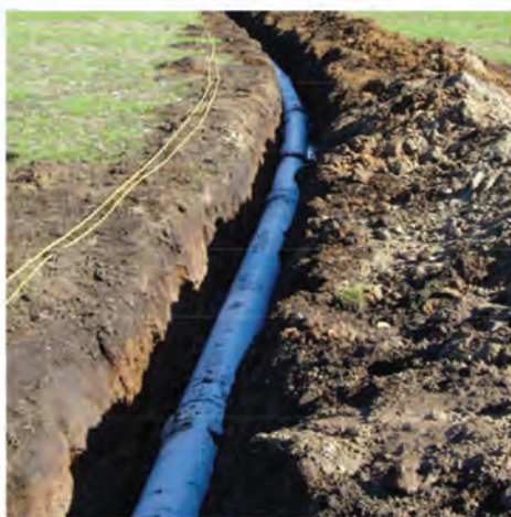
Figure 7.10: Curved pipeline installed ready for backfilling.
