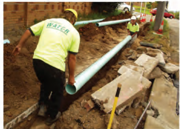
Figure 7.3: Faster installation is possible especially on congested sites owing to the pipes light-weight nature and minimal jointing force required when using ApolloBLUE™
