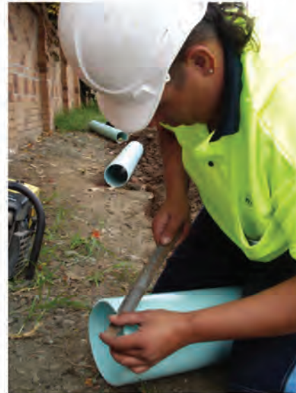
Figure 7.7: Chamfering the cut end of an ApolloBLUE™ pipe by hand.
