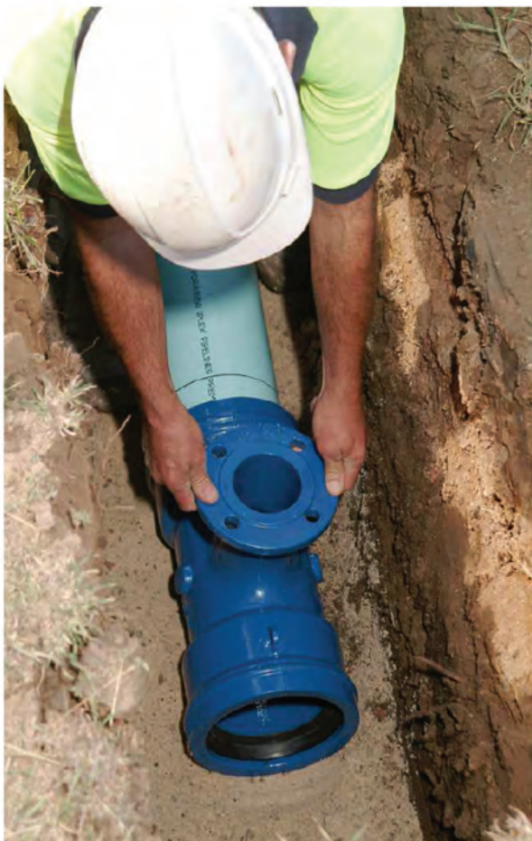
Figure 4.2: Polymeric coated DI hydrant tee – note witness mark on the ApolloBLUE™ pipe spigot to ensure full insertion is achieved when joining.
