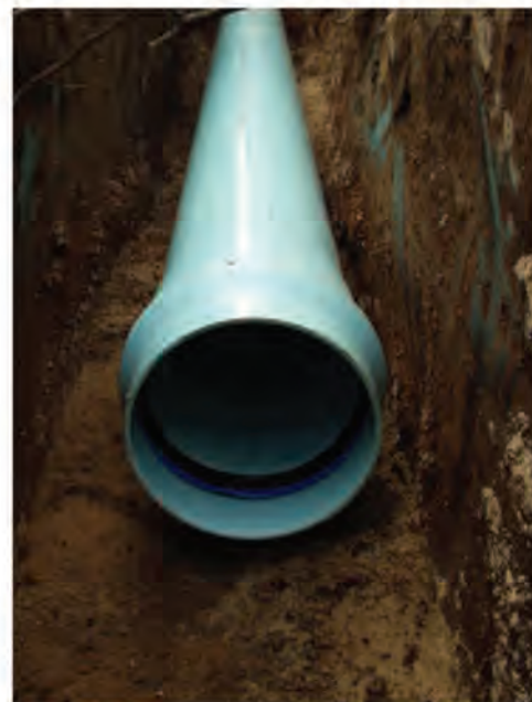
Figure 6.1: ApolloBLUE™ should be installed in the same way as other PVC pipes that are fully surrounded and embedded in a compacted granular material with “bell holes” for the sockets.
