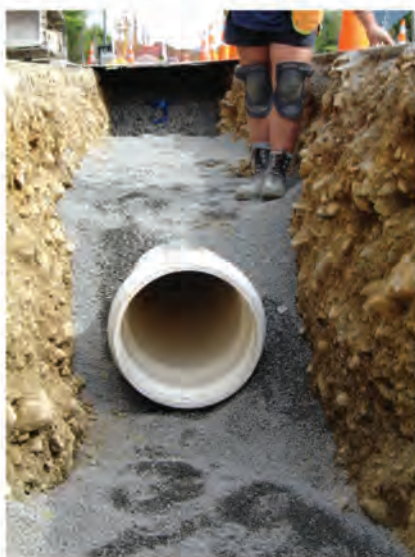
Figure 7.3 – Imported embedment material is well compacted around the pipe for support.
