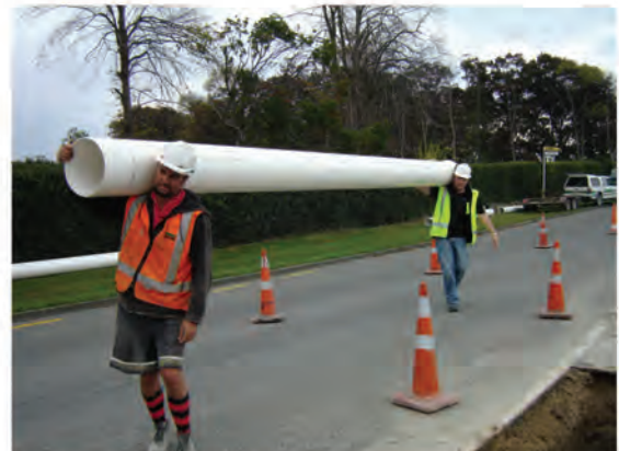
Figure 1.3 – The light weight nature of PVC pipes allows ease of handling during installation.
