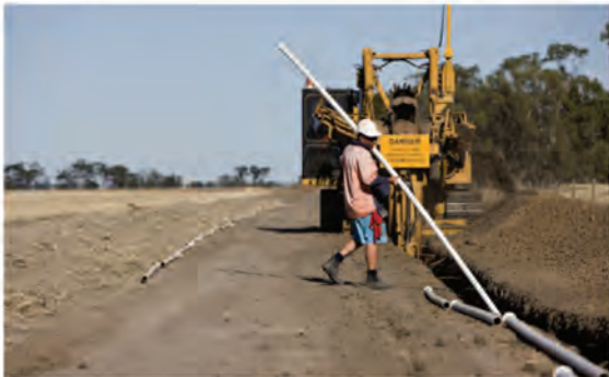
Figure 1.1 - PVC irrigation pipe installation
