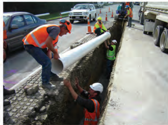
Figure 1.2 – Potable water PVC-U pipeline installed in roadway.
