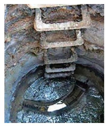
Figure 1: Corroded iron steps in a conventional maintenance hole.
