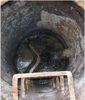
Figure 2: Sulphuric acid corrosion in a conventional maintenance hole.
