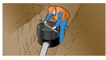
**O3** Adjust the pipes to the required position. The adjustable pipe connector enables an angular deflection of 7.5° from the centre line in all directions.
