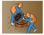
ring. Remove the lid from the cap and apply GATIC<sup>®</sup> sealing compound liberally to all vertical and horizontal seating surfaces of the lid and assemble on the cap.
