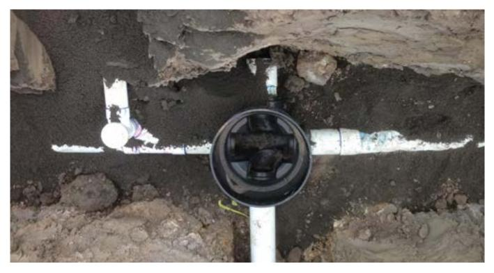
Figure 3: Iplex EZIpit® 425 MS base with 4 way 'x' profile channel and PVC DWV pipe.
